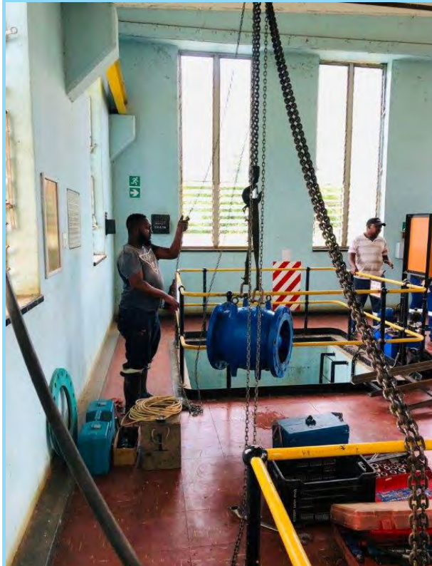
Repairs of non-return valves within the Ebenezer Scheme for pump protection and control
