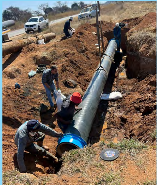
Pipe repairs of 500mm pipe near Tompi Seleka. The pipe was dilapidated resulting in high water loss
